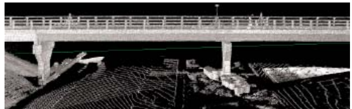
Photo of one of the surveyed bridges.
